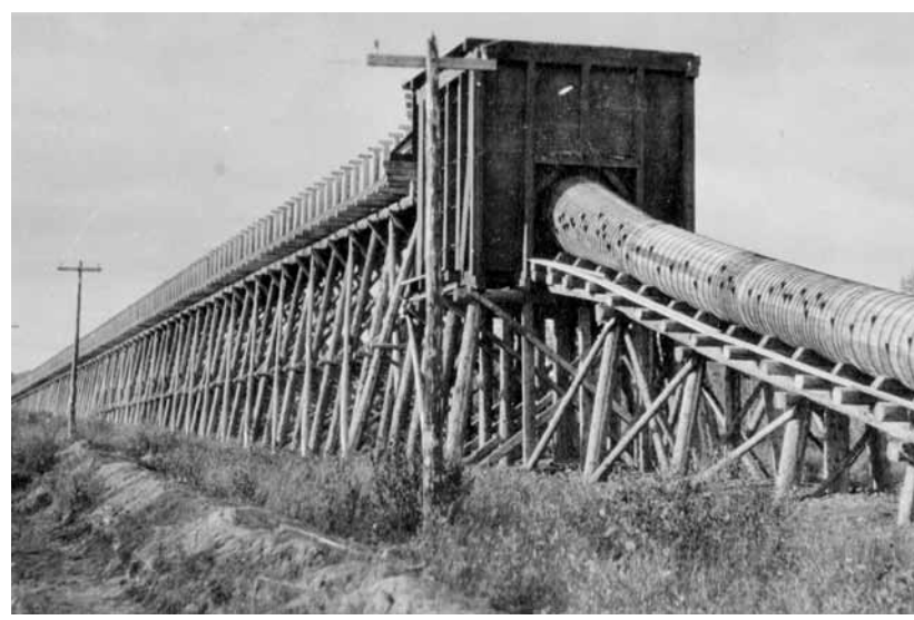
Flume, pressure box and wood stave siphon. YA, Emil Forrest fonds, 80/60 #108
